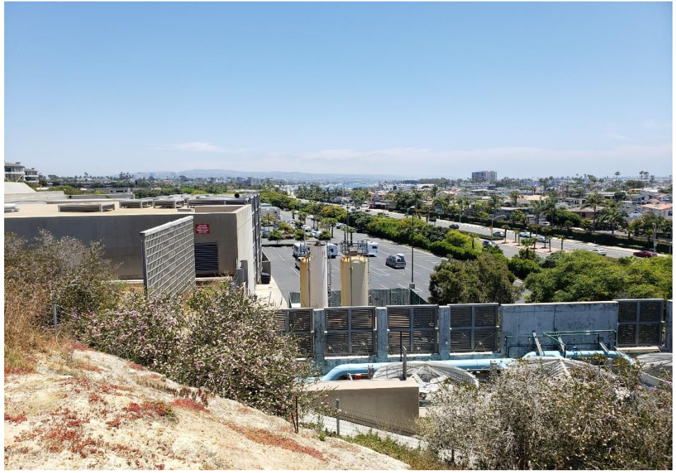
Photograph 7: Looking east away from the site at the Hoag Child Care Center.
