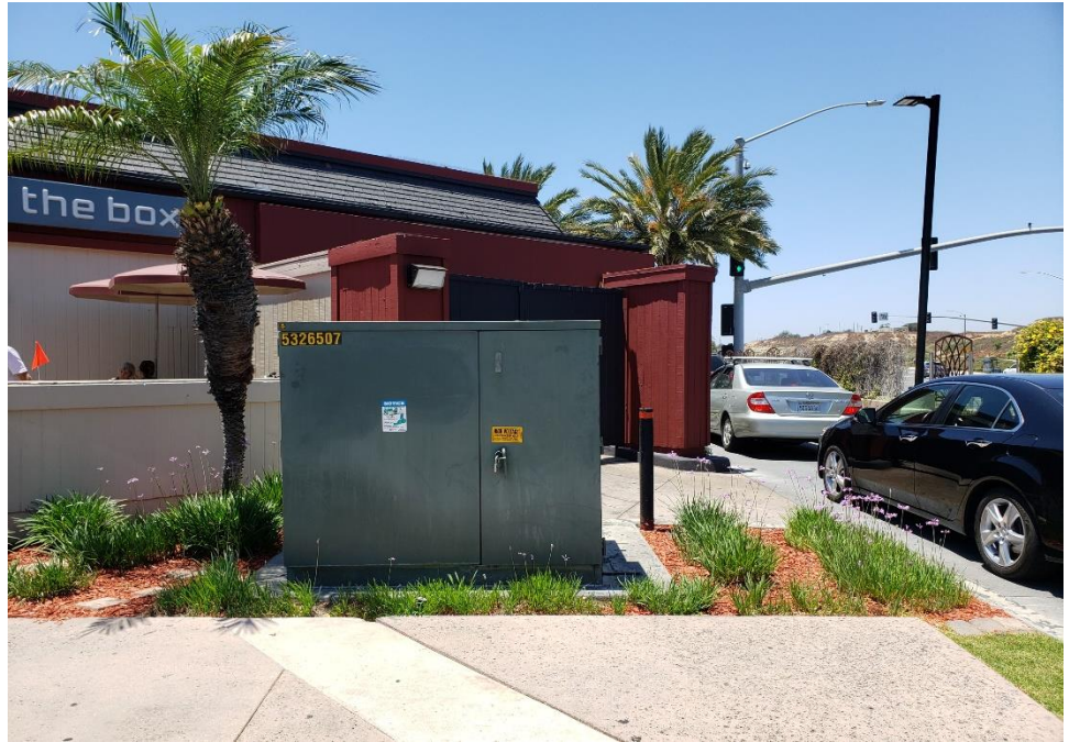
Photograph 3: View of pad-mounted transformer located at the northeast corner of the Jack in the Box Property, adjoining the site to the south.
