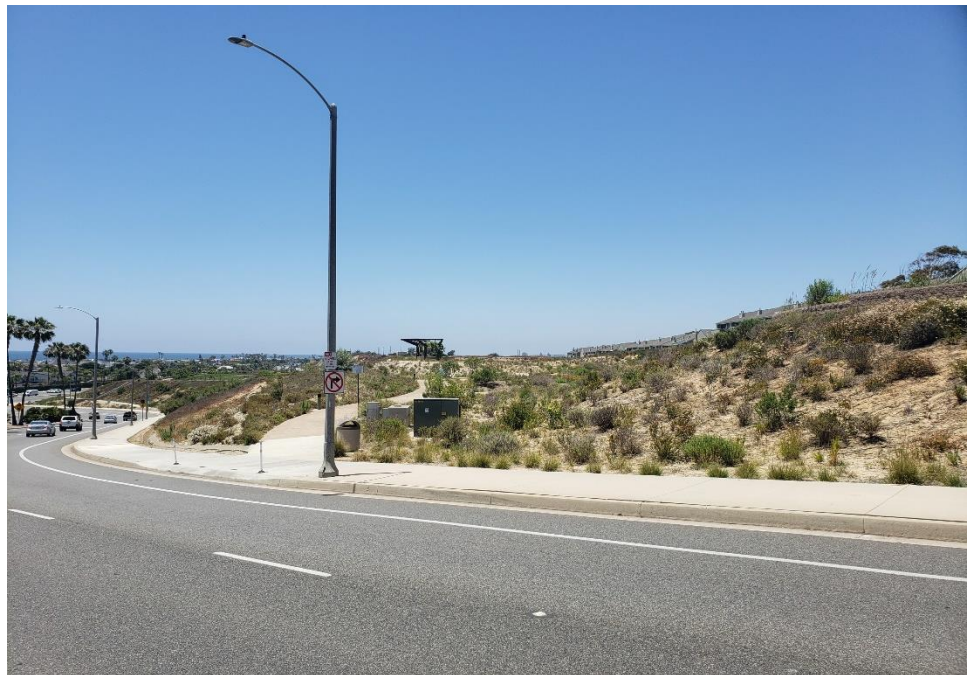
Photograph 4: View of pad-mounted transformer in eastern portion of Sunset Ridge park, northeast of the site.
